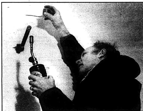
Fred Denn repairs pipes where they had burst and flooded the house the week before. Photo by Kelly Wells
