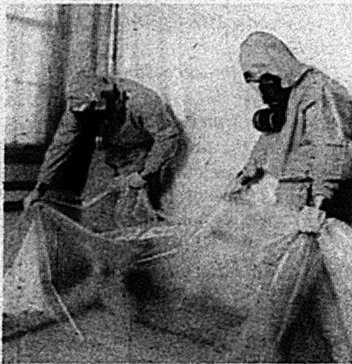
Workers removing asbestos.
