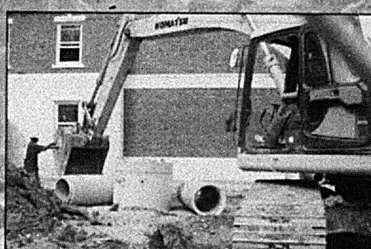
With his coworker's aid, Max Gill of Stilley Company maneuvers sections of storm drain. In order for the Potomac River residence hall ready for occupation, proper drainage systems must be in place.
